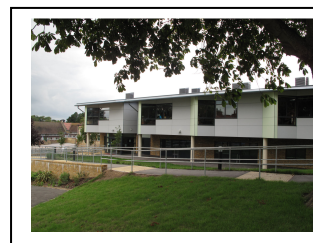
Balfour extension completed in 2009
